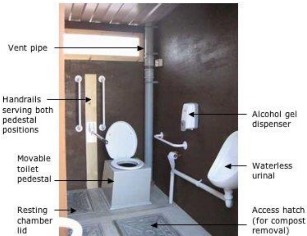
Interior of a full access twin-chamber urine-separating compost toilet, incorporating a waterless urinal, powered venting, and alcohol gel for hand-cleansing (Picture courtesy of Natsol Ltd).
